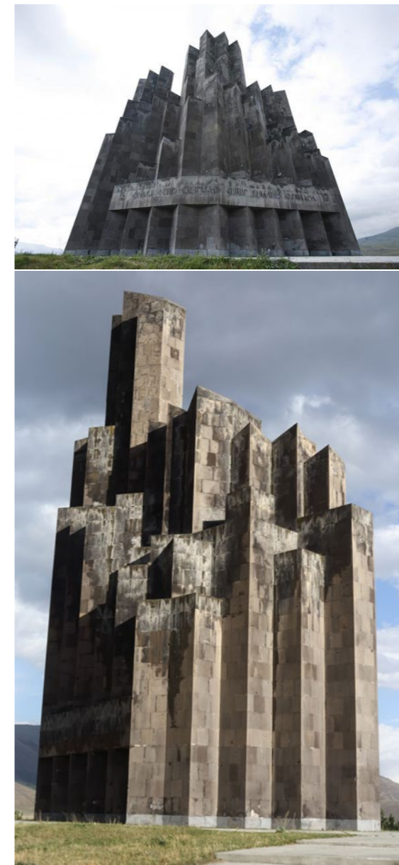
The northern facade
