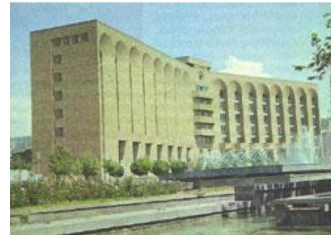
3rd Government Building, Yerevan, T.Gevorgyan, V.Housyan, 1980
