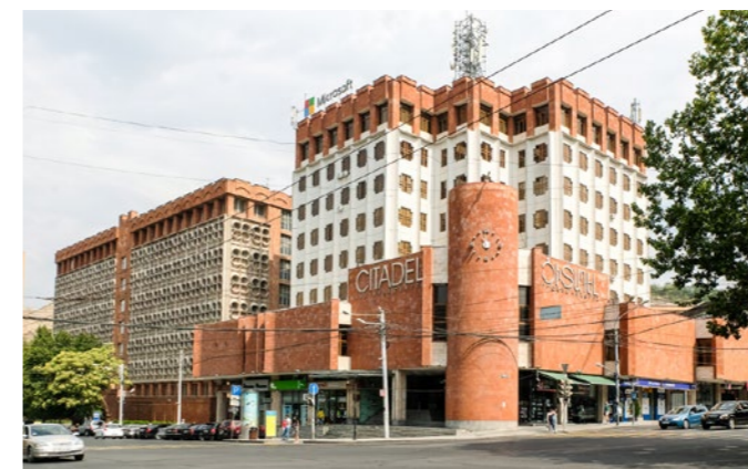
'Citadel' Business Centre, Yerevan, A.Aghalyan, 1990s
